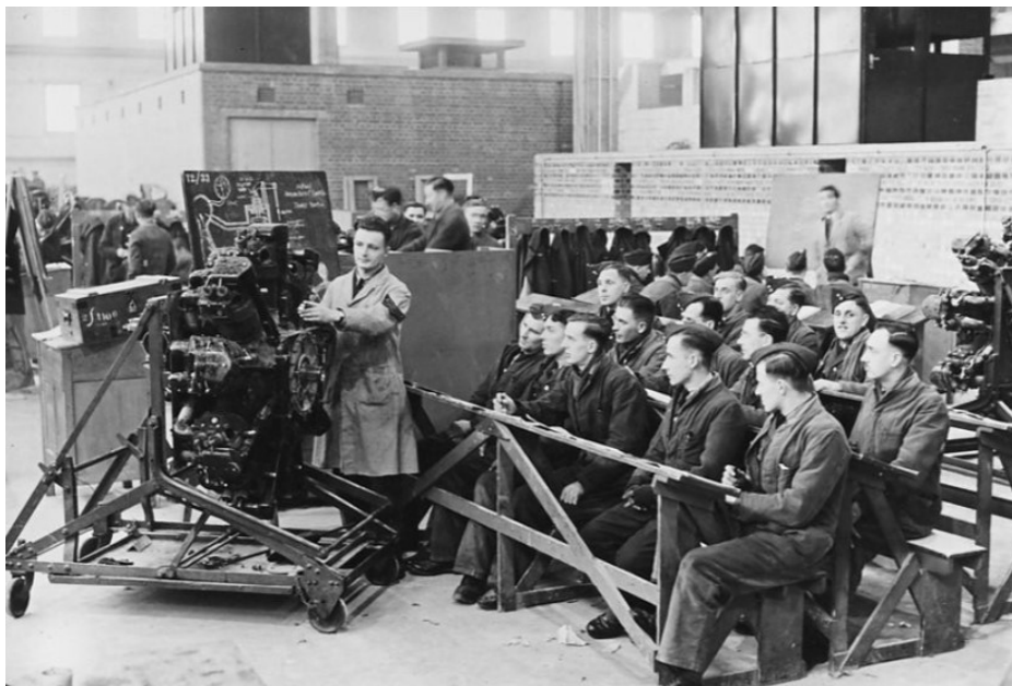
Engineering lesson on a Bristol Mercury radial piston engine
