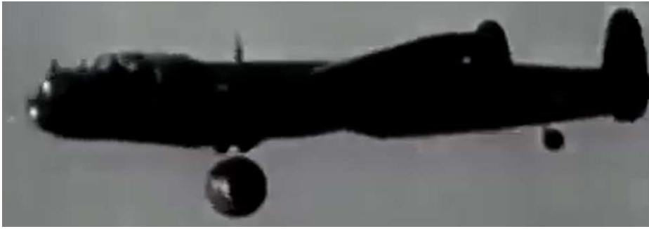
Lancaster ED817 dropping a wooden cased Upkeep at Reculver
